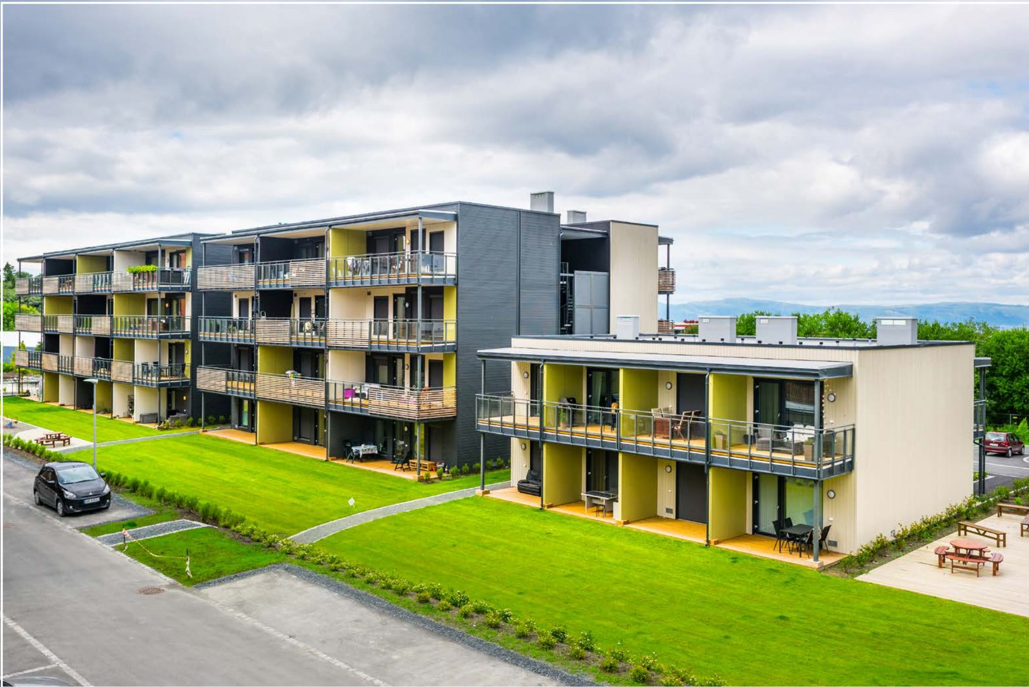
Miljøbyen Granåsen, Trondheim, Norway – passive construction
